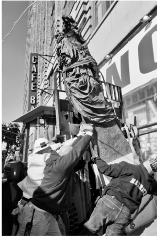
NYRPA moved from Crossroads School of the Arts & Sciences to the World Trade Center entry & Nino Vendome site by Howard Silversmith. Photo by: Peter Danello, Jr.
